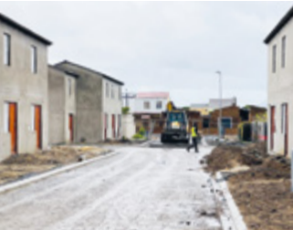
Taking shape: The infill housing project in Gatesville is going according to plan. It will provide 135 affordable housing opportunities to residents of the Pooke se Bos informal settlement. The total cost of the project is R45 million, which includes civil and electrical works, landscaping and top structure construction.
